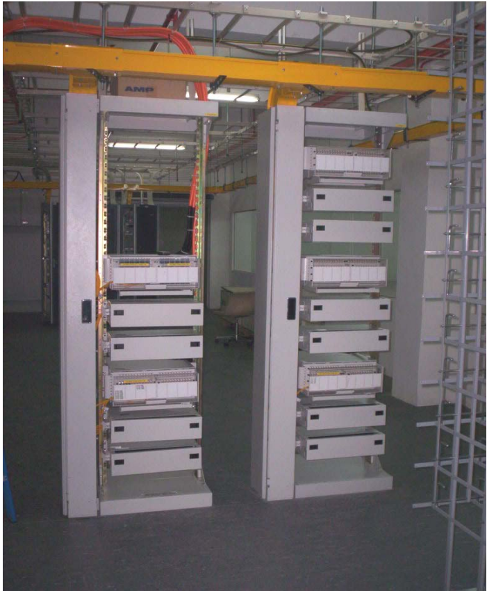
FIBRE TERMINATION & DISTRIBUTION SYSTEM (FTDS)
